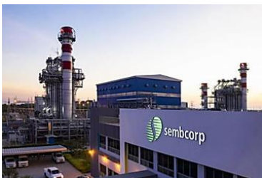
Temasek is right to abandon Keppel for deal with Sembcorp Aug 17, 2020
